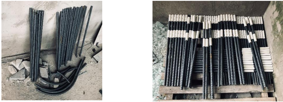
Figure 3. Preparing steel bars.
