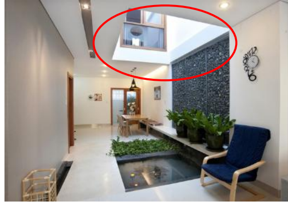
Figure 3. Architectural slab openings.
