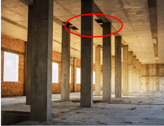
Figure 2. Technical openings adjacent to columns.
