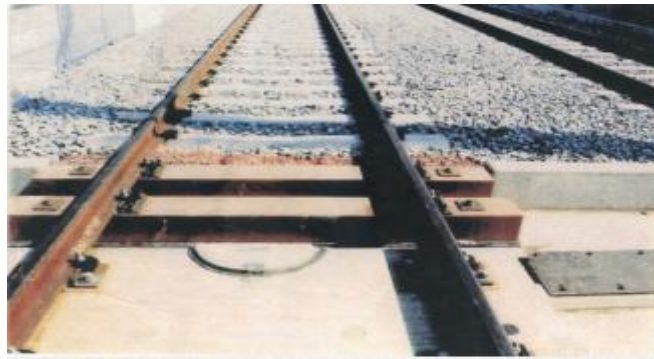
b) Ballasted/Ballastless Track Elastic Sleeper Transition
