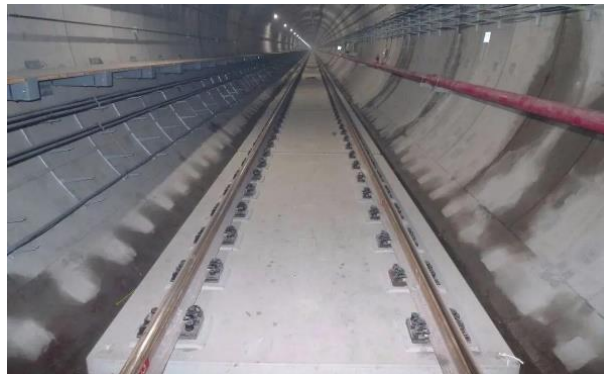
Fig 1. Embedded block track [8].
