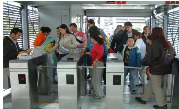
b) AFC system at the station
