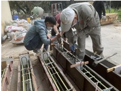
Figure 6. Compacting and pouring concrete process.
