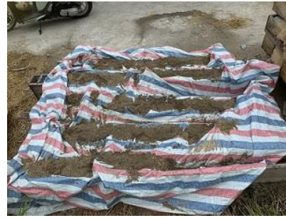
Figure 7. Curing beam specimens after casting with moist sand.
