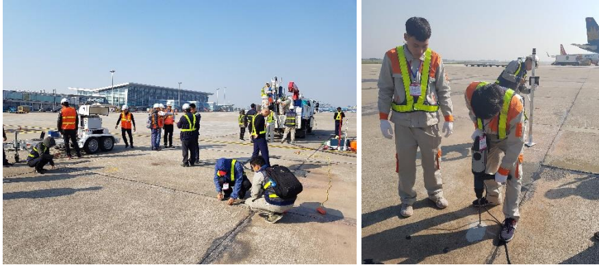
Figure 6. Determine the location of guide pipe for polymer grout injection.
